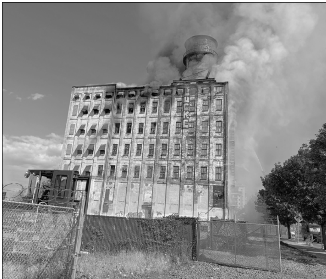
116-year-old 8-story former warehouse on fire.
